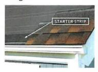
GAF Lifetime Algae Resistant architectural shingles installed per manufacturer's current specifications, guidelines & High Wind Nailing Pattern.
